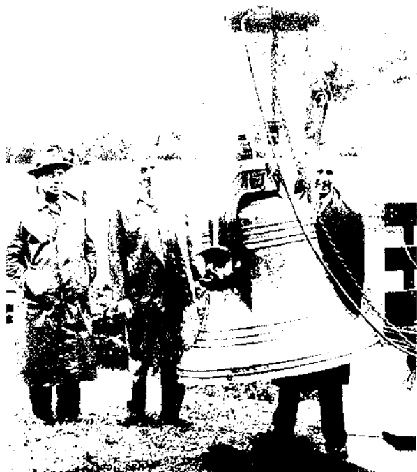
Unloading our church bell, given by the Thomas Lencis in 1958. Supervising the operation are Sexton Pieter Van Kroonenburg, George Simson and Dr. David Barnwell. The bell was hoisted into the tower after tearing out part of the vestibule ceiling.
